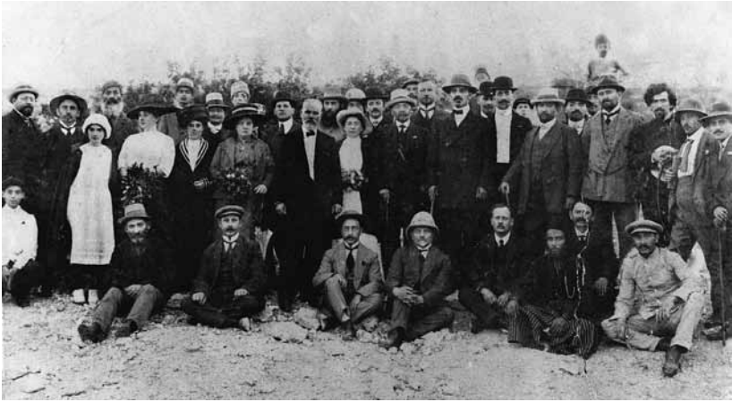
Laying the cornerstone for the “Technikum” (later, Technion), 1912
