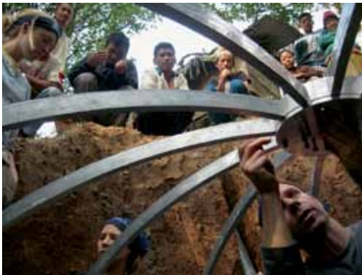
Technion’s Engineers Without Borders: Helping the world
