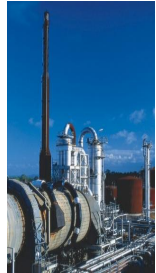
Queensland Australia Syn-Crude Plant
