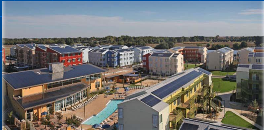
UC Davis West Village - 4,000 kW Solar PV System
