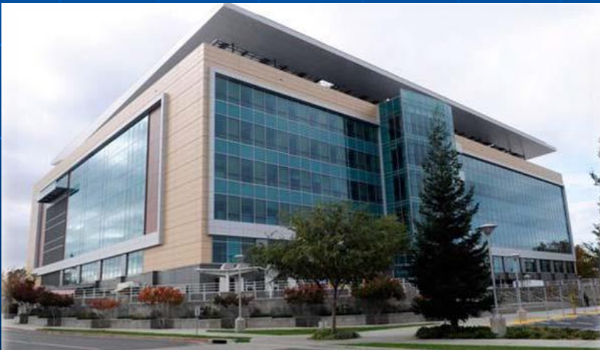
Dept. of Motor Vehicles HQ - 428 kW Solar PV System
