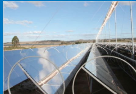
Close-up of compact linear Fresnel reflectors focusing sunlight onto a receiver.
