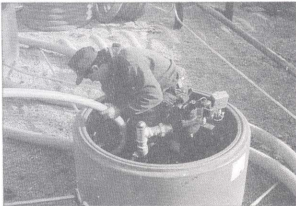
Flexible Enviroflex primary piping reduces installation time by 50%.
