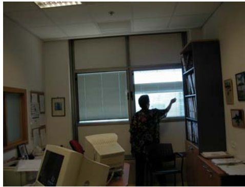
Southern, eastern and western façade windows with embedded blinds
