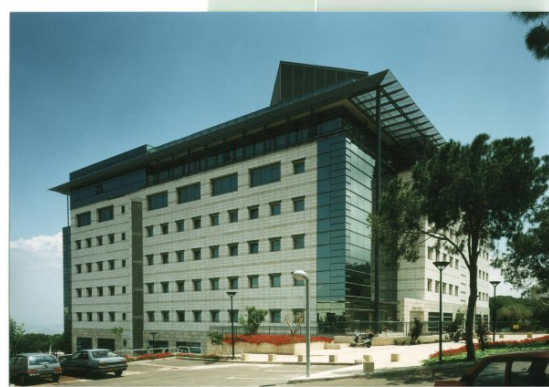
Western and southern facades
