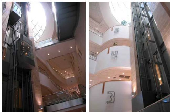
Atrium roof –view from below
